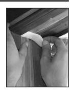
5. The metal clips are to be positioned against the jamb, approximately 4" down from the head jamb and 4" up from the sill. Attach these clips into place using the supplied #7 x 7/8" screws. Clips should be installed level and tight to inside stop.
